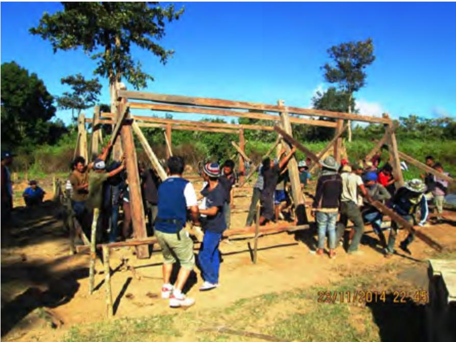
Very successful was the combination with skills training on construction: Participants of the training constructed the floor, they produced the needed brick blocks, and they set up the roofs.
